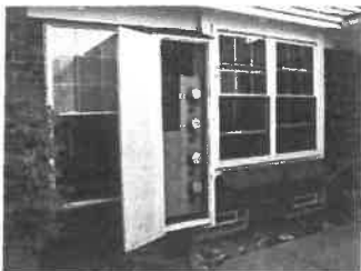
Meter Box Outside
