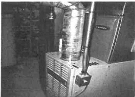
Furnace Electrical and Gas Shut-Off Points Gas – Black pipe and red handle.....Electrical - Looks just like a light switch
